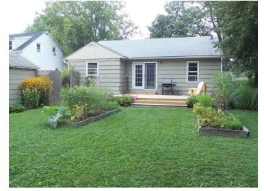
are in generally good condition. All doors were opened and they operated freely. The deck(s) appear to be constructed from pressure treated wood – a rot resistant material.
