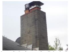
be in good order. The installation of the roofing materials has been performed in a professional manner. Installation details look neat and trim. Rain caps and vermin screens have been installed on the masonry chimney flues. The gutters are clean. A plumbing vent pipe was observed to penetrate the roof at normal height and in good condition.
