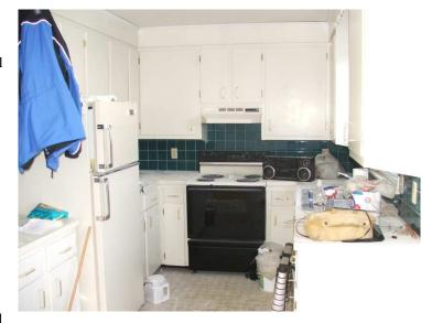
• **Safety Issue, Repair:** The electric range top is lower than the counter. This can burn the counter. It should be adjusted up according to the manufacturer recommendations. A qualified appliance repair technician should perform this work.
