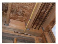
The spans of all observed joists and rafters appear to be within acceptable limits and no appreciable movement was noted when floors were 'bounced upon'. They were observed to be clean and free of rot with only minor, typical cracks. The carrying beams and support columns were reasonably straight and in good condition with no significant rust or rot. The exterior plane of the roof was even and flat.
