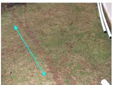
• Monitor: An exterior 'Perimeter Drain' or 'Footing Drain' apparently exists. Recommend capping the exit pipe (usually found at the low point on the lot) with a vermin screen. Recommend periodic flushing with water and monitoring the end of this pipe.
