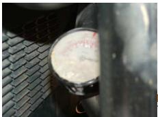
Repair: A leak has damaged the gage. Leaks at heating equipment should be repaired promptly to avoid damage to the equipment or to the building and to assure reliable system operation.
