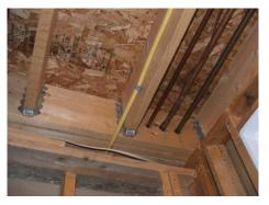
The spans of all observed joists and rafters appear to be within acceptable limits and no appreciable movement was noted when floors were 'bounced upon'. They were observed to be clean and free of rot with only minor, typical cracks. The carrying beams and support columns were reasonably straight and in good condition with no significant rust or rot. The exterior plane of the roof was even and flat.
